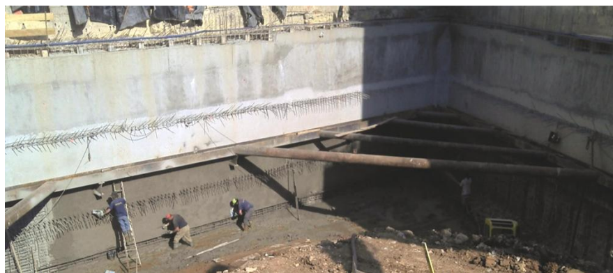
Figure 15: View of the SMW with the steel waler beams, the internal struts and the concrete wall, after Peixoto et al. (2012c)
