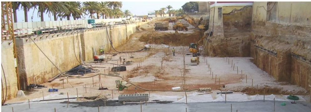
Figure 14: View of the excavation, after Peixoto et al. (2012b)
