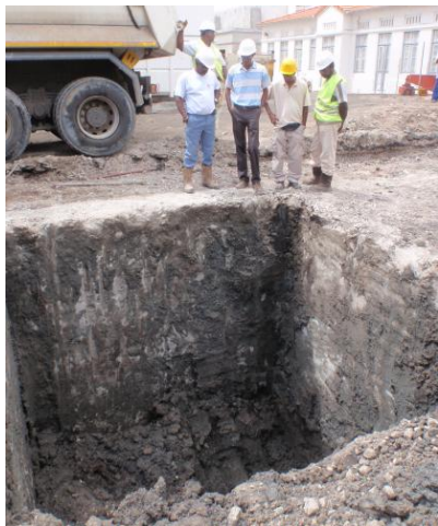
Figure 34: Excavated Geomix caisson, after Benhamou and Mathieu (2012)
