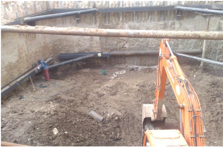
Figure 13: View of the excavation after the execution of the second level of struts, after Peixoto et al. (2012a)
