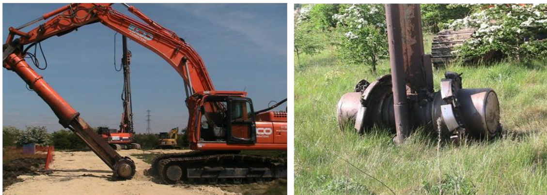
Figure 8: The ALLU® system used in the ground improvement treatment sections (Al-Tabbaa, 2012)
