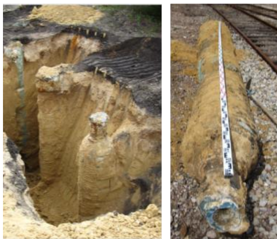
Figure 35: Excavated soil-cement columns 1 month after construction, after Guimond-Barrett et al. (2012a)
