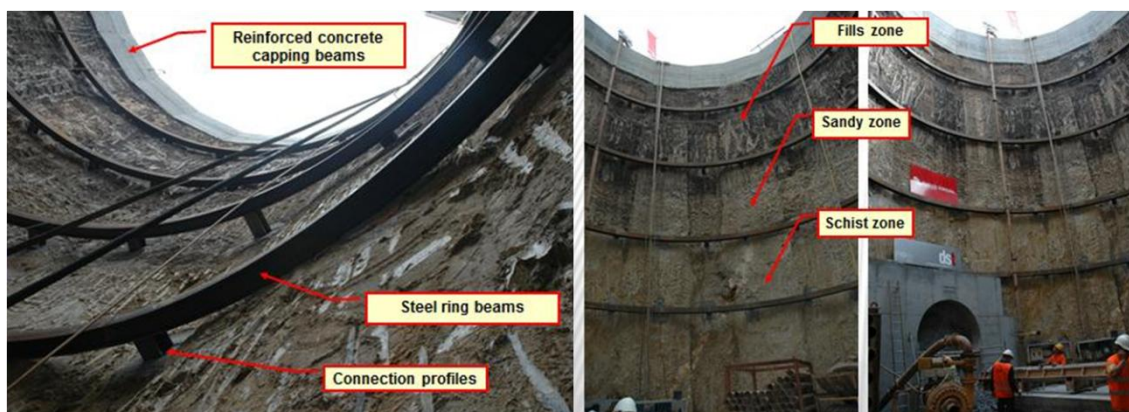
Figure 17: Inside view of the right bank shaft after excavation, after Pinto et al. (2012)
