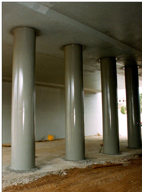
Estacas-Pilar (após acabamento final)/Pile-Pillars (after finishing work)
