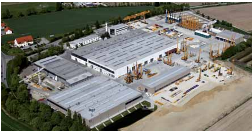
The Aresing plant (above). Works extension at Klemm in Drolshagen (right)
