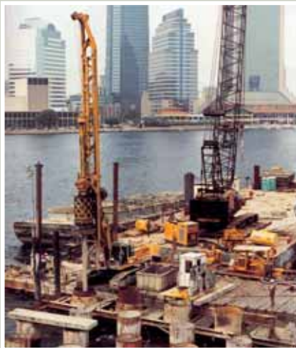
Difficult: the Acosta Bridge in Jacksonville
