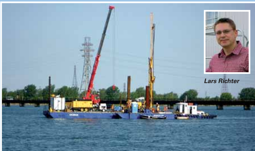
Drilling from pontoons into rock: constructing bridge foundations near Montreal. The first office of the site team headed by Martin Pielmeier (second from right) had more of a kitchen feel to it.
