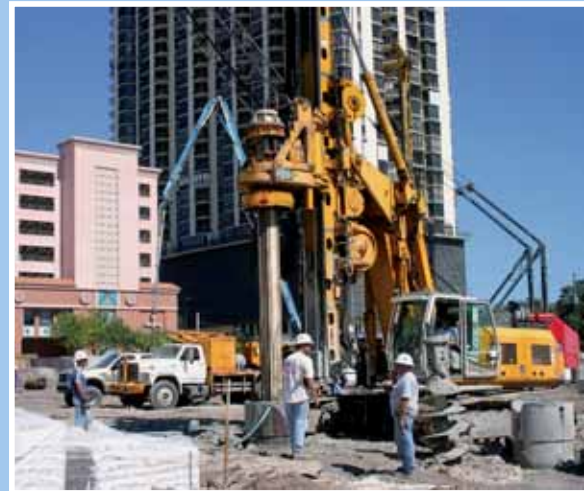
Coastal Caisson working in Tampa, Florida
