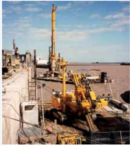
Remediation works with a Bauer BG and UBW in the port of Buenos Aires
