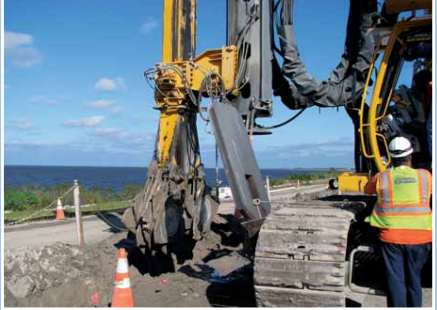
Redevelopment of the Hoover Dike around Lake Okeechobee; see also picture below
