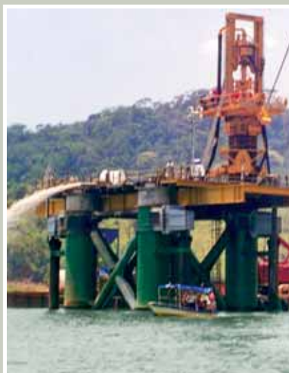
Reverse circulation drills were deployed on the Chiapas Bridge foundations in Mexico.
