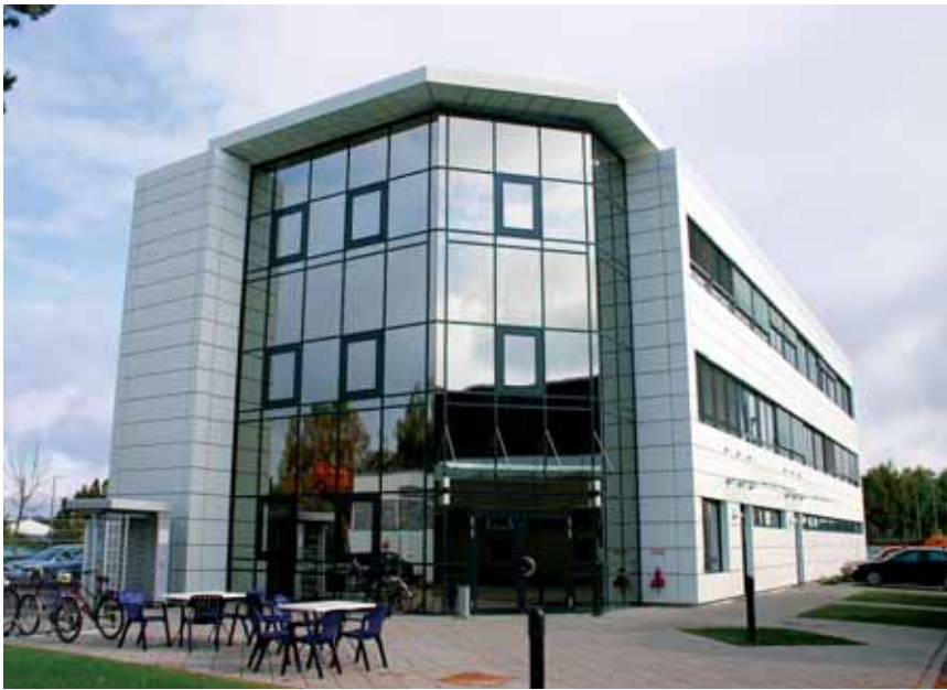
New office building at the Aresing plant
