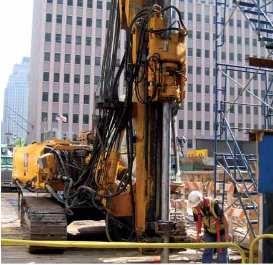
Jet grouting by Bauer machinery in downtown New York
