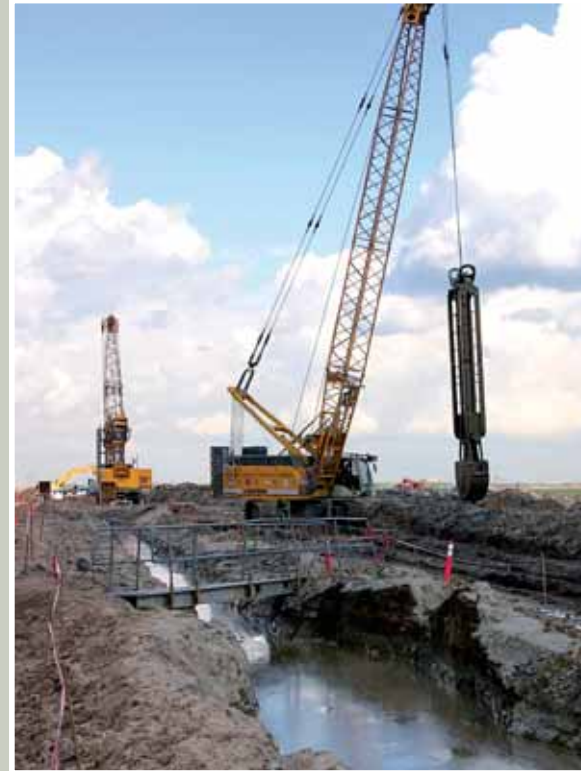
A grab-excavated cut-off wall protects a river against pollution from oil mining.
