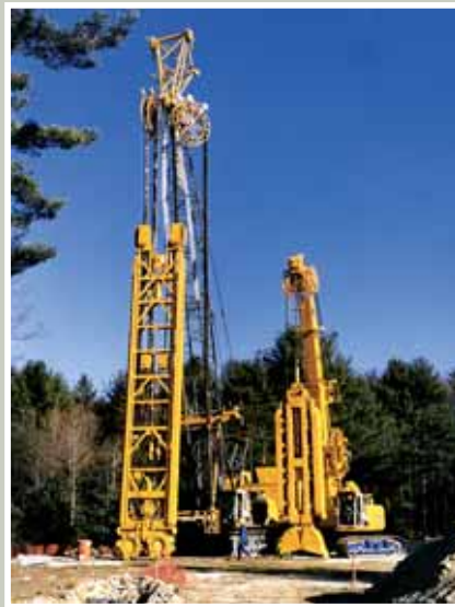
Successful: remediation of the Hodges Village Dam
