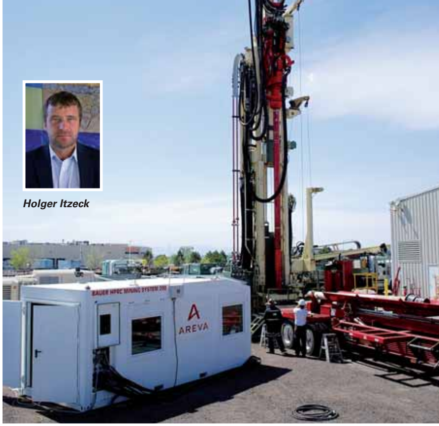
Deployment of specialist foundation engineering methods in exploration and mining
