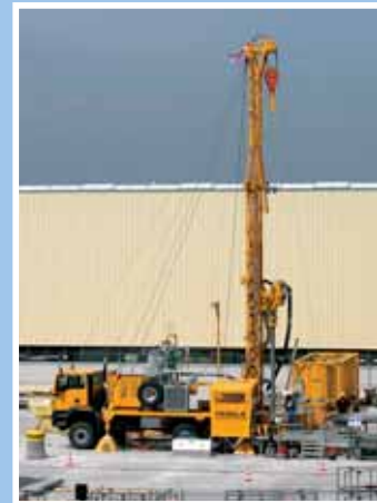
The "anchor casing tour" at the drilling site in Edelshausen was executed with a Prakla drilling rig.
