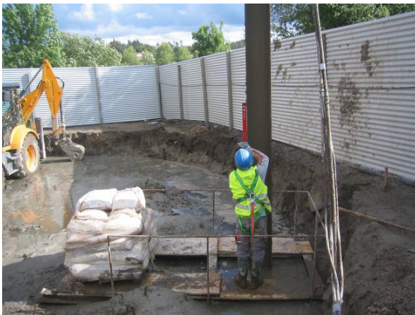
Installation of reinforcing steel beam
